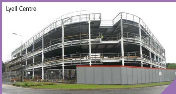
Ongoing works at the Lyell Centre include excavations for foundations, substructure and drainage works, structural foundations and a temporary site access bridge.
